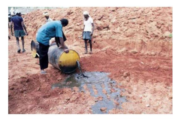
An internal boundary was marked for 2mtrX15mtrs, in orderto accommodate the 10kilolitres of sludge, thus making a small pit. The sludge from each barrel has been transferred inside the small pit.
