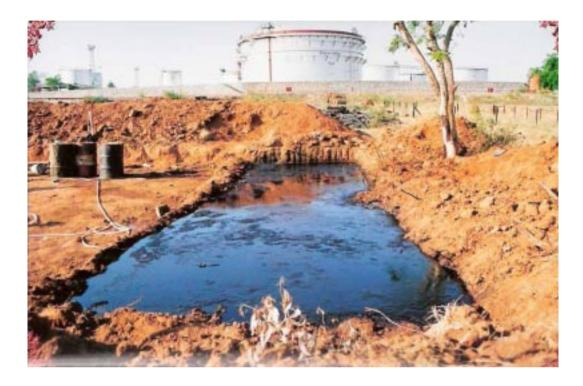
The sludge which was dumped from the barrels has been evenly distributed through out the pit with the help of crowbars, and long handle shovels. After this process, the sludge was levelled, and was made ready for Bio-remediation.
