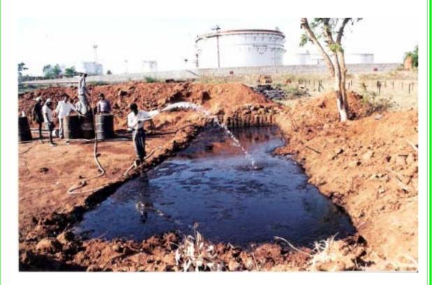
After the leveling of the sludge fresh soil (clay) was sprinkled on the surface of the sludge through out the pit, upto a height of 2 inches. This was mixed thoroughly by manual process using long crowbar, so that the sludge and soil mixture is formed.
