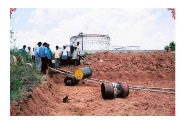
As per the instructions of Karnataka State Pollution Control Board, the quantity 10kilolitres is ear marked for the trial. Since the sludge is stored in barrels, a convenient method of transporting the barrels to the pit has been taken up by a ramp in one corner. By this method, all the 50 barrels were rolled inside the pit manually. Since these barrels were sealed, there was no leakage at any place on the way.
