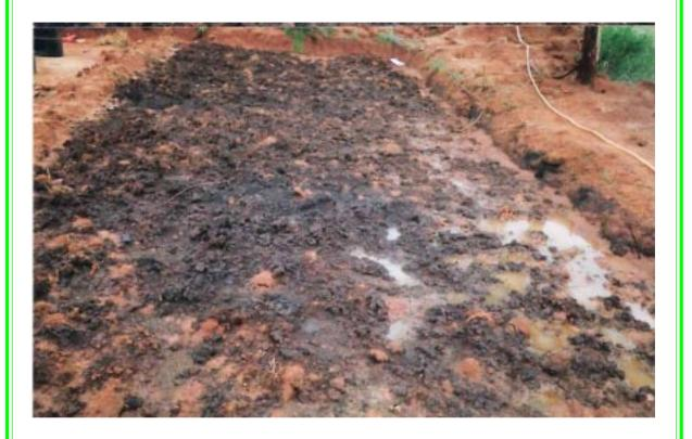
It is highly essential to maintain moisture in the pit. Hence spraying of water was consistently done on a daily basis. A dosage of 100 litres water spray in the morning and 100 litres in the evening was maintained, on the surface of the sludge through out the pit to keep the sludge wet.
